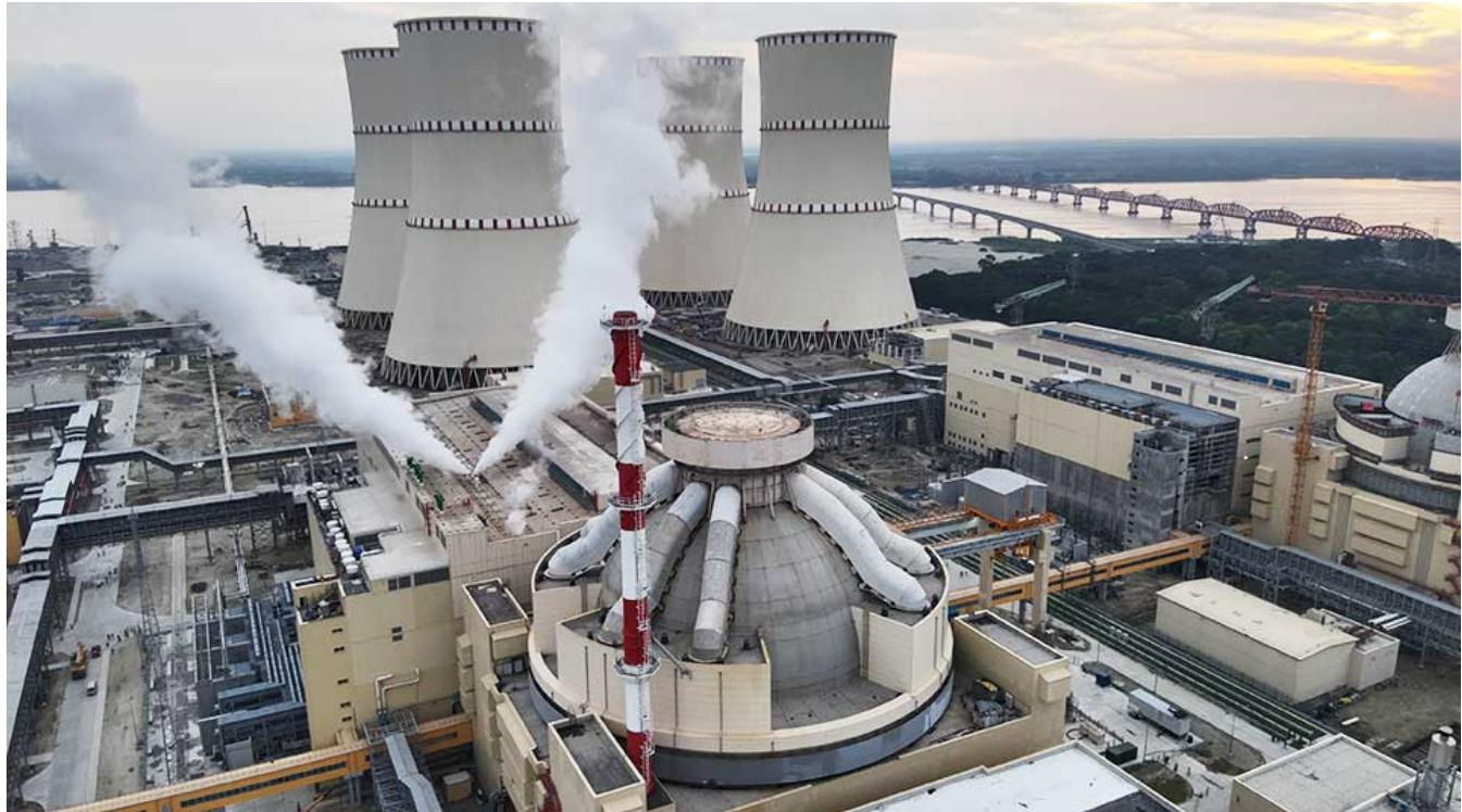
One of the key stages of cold and hot functional tests has been completed during a set of commissioning activities, such as blowdown of the fresh steam pipelines in the turbine compartment at Unit 1 of the Rooppur NPP. The results have proven that the unit's steam pipelines are available for supplying steam to the turbine
