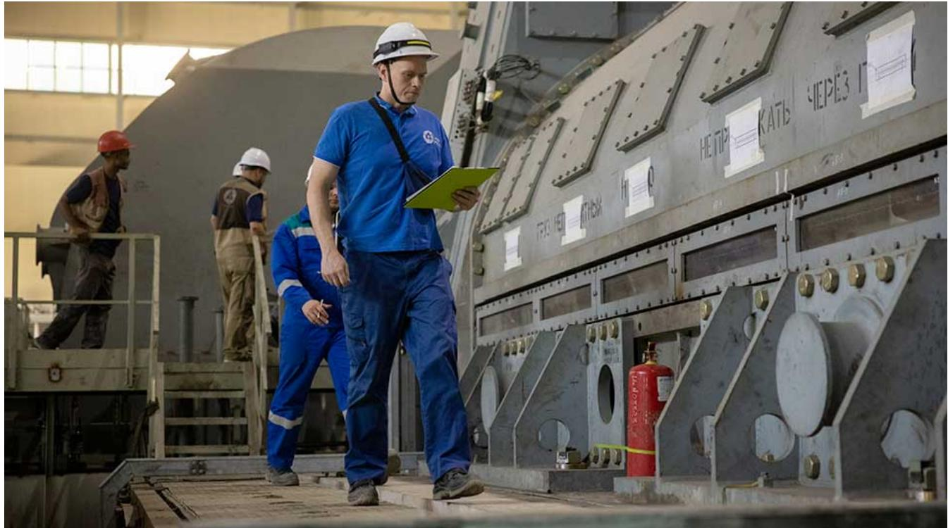
An important and final stage of the turbine installation has been completed at the first unit of Rooppur Nuclear Power Plant. This resulted in the turbine set placement on the barring gear. During the tests, the turbine shaft was rotated at a slow speed.
